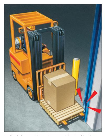
Loading dock sectional door tracks are especially vulnerable to frequent damage. Pipe bollards cannot completely protect against the traffic and high activity typical of the loading dock environment.
